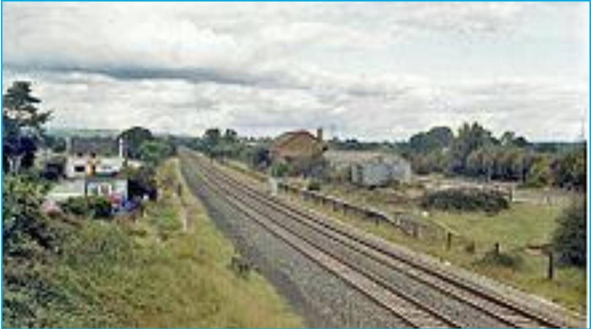
Cullompton station as it was in 1984, looking north from Station Road bridge – showing the space created in the 1930s for platform loops off the main line. The photograph may distort matters, but it appears that the main line has been slewed partly into the formation of a loop line.
